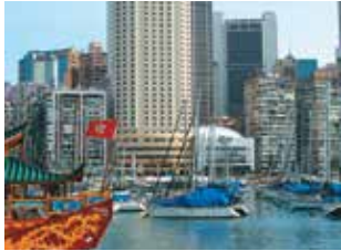
The Excelsior, Hong Kong
